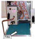
These systems have a feature called True Sense filter detection. This feature reads the change in static pressure caused by the filter accumulating dirt. At a preset time every day, or at the factory default setting of 1:00 PM, the system will take a reading and record the change in static pressure. The "clean or replace filter" message will pop up when the filter is full.
