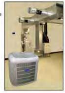
If the zoning system will not run or shuts down intermittently, and EXCESS STATIC PRESSURE appears in the LAST 10 SYSTEM EVENTS, this indicates that the controls have increased the RPM of the indoor fan to MAXI-MUM in an unsuccessful attempt to maintain the equipment minimum airflow rate against a high ductwork static pressure loss.
